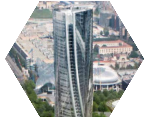
Milan, Italy CITYLIFE SPA Design and installation of a G-iron shield on walls and floor, and of shielding cable trays
