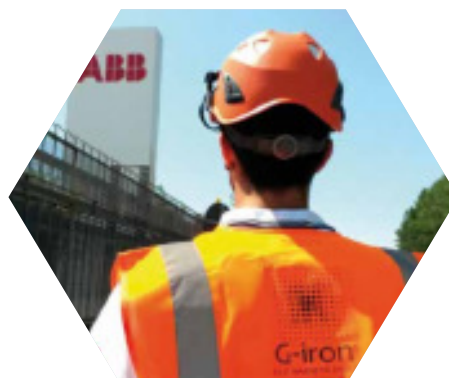
Milan and Arezzo, Italy ABB Installation of a shielding system serving the purpose of protecting employees on their workplace
