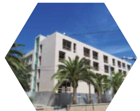
Lorca, Spain GUARDIA CIVIL The shielding system was designed and installed inside an HV/LV substation
