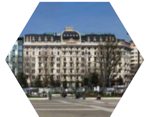
Milan, Italy HOTEL EXCELSIOR GALLIA Shielding of a substation to protect the conference room
