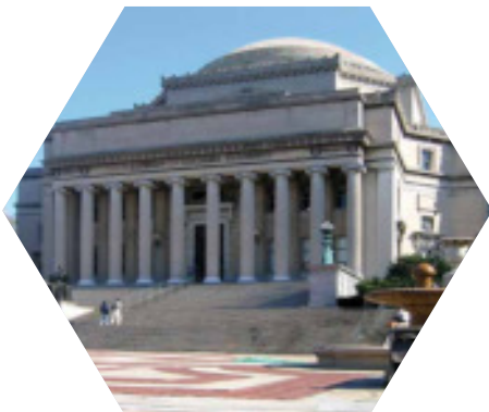
New York, USA COLUMBIA UNIVERSITY G-iron Flex™ tested in view of future installations of shielding systems in certain areas of the building
